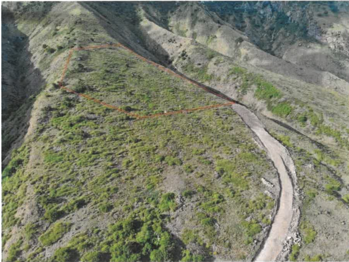
Figure 1: Aerial View of the RE Phase 3 Site in Giles Quarter
